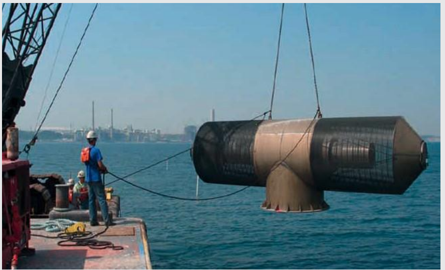
JOHNSON SCREENS® Passive Screen Installation for WE Power at Lake Michigan
